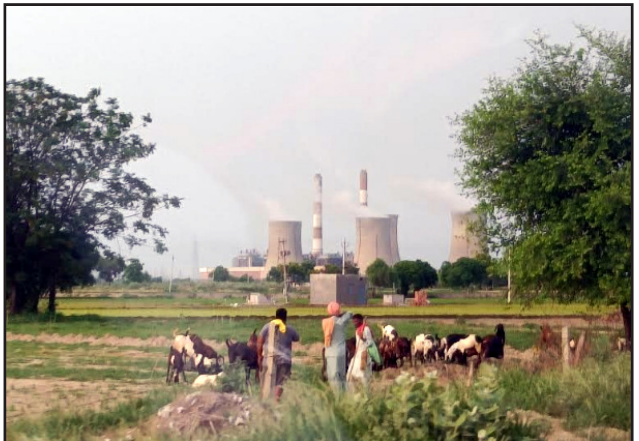
Shri Guru Hargobind Thermal Power Plant situated Lehra Mohabbat (Bathinda) spread over 1025 Acres area, and having generation capacity of 920 MW, run by coal & furnace oil, serves huge area of Punjab/ Sunil Kumar Gund
